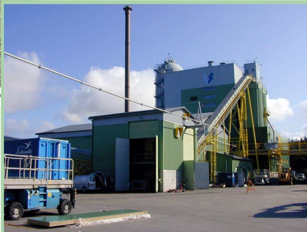
Power plant of Kokkolan Voima Ltd. Reed canary grass chop is transported pneumatically to the boiler via the pipeline on the left. (Photo: Timo Lötjönen, MTT).
